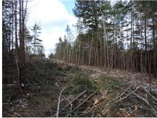
A new road to the new cut in photo above
